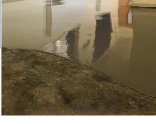
**SETCRETE LEVEL-SMART** is designed for preparing sound internal subfloors prior to the installation of new floorcoverings and can be applied at thicknesses from 2-30mm. It is particularly suitable for direct application over old adhesive residues (such as bitumen and carpet tile tackifiers) without the need for priming. Its fast setting characteristics enable a walk-on time of just 90 minutes and new floorcoverings can be installed from 4 hours.
