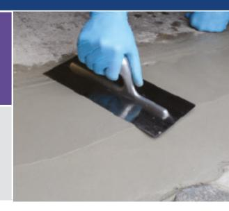
**SETCRETETM CONCRETE REPAIR** is an easy to use, single component, Polymer Cement Concrete (PCC) mortar for the non-structural repair of damaged or worn concrete. It is suitable for use on both internal and external applications and can be applied to horizontal and vertical concrete surfaces.
