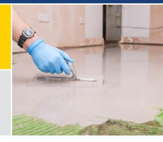
**SETCRETE<sup>®</sup> UNIVERSAL** is suitable for use over a wide range of absorbent subfloor types including sand/cement screed and concrete. It is also suitable for use over non-absorbent subfloors such as ceramics, granolithic, terrazzo and quarry tiles, providing they are sound, well adhered and suitably prepared.
