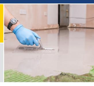
**SETCRETE™ UNIVERSAL** is suitable for use over a wide range of absorbent subfloor types including sand/cement screed and concrete. It is also suitable for use over non-absorbent subfloors such as ceramics, granolithic, terrazzo and quarry tiles, providing they are sound, well adhered and suitably prepared.
