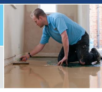
**SETCRETE** RAPID SET 30 utilises the latest advances in cement technology to achieve a walk-on time of as little as 30 minutes and its rapid drying formula means that new floorcoverings can be installed from just 2 hours. As it is a water mix, it also offers the advantages of being economical and latex free.
