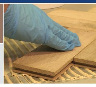
**SETCRETE FLEXIBLE WOOD FLOORING ADHESIVE** is a highly flexible adhesive suitable for the installation of engineered or solid plank, wood block and wood strip flooring. It is quick setting and develops a high bond strength. It is also suitable for use over underfloor heating systems.
